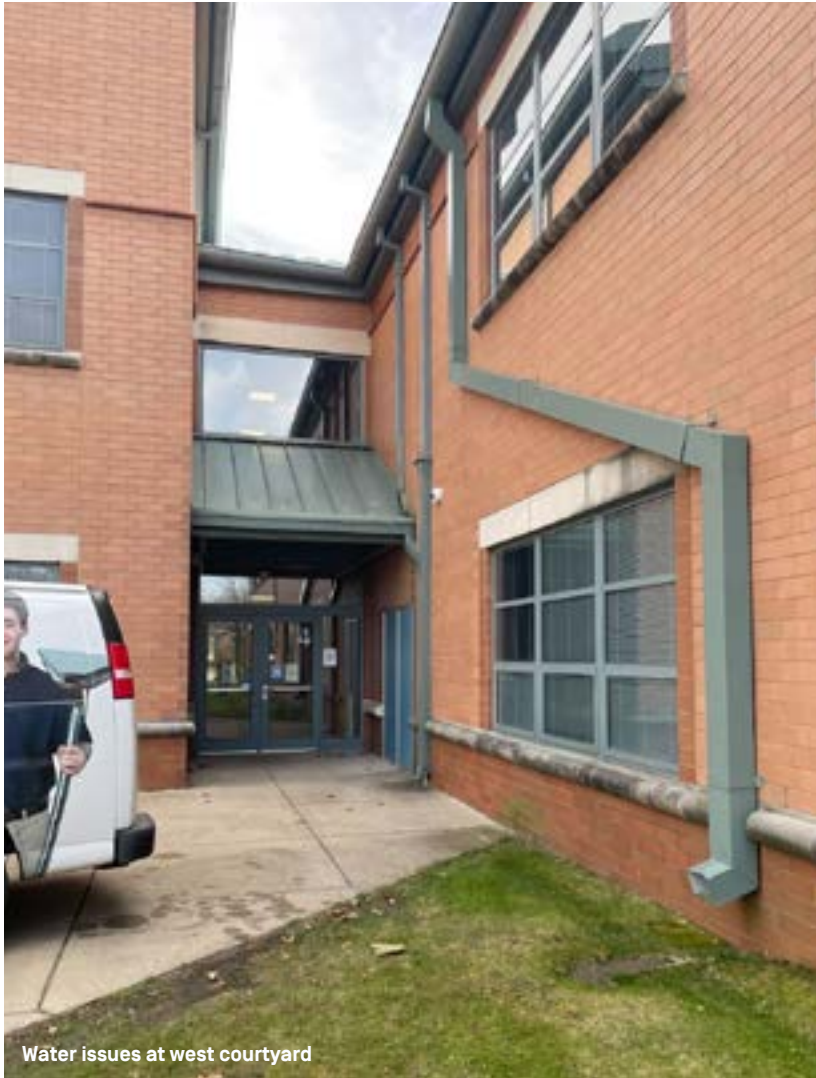
Limestone sills to be cleaned and sealed
